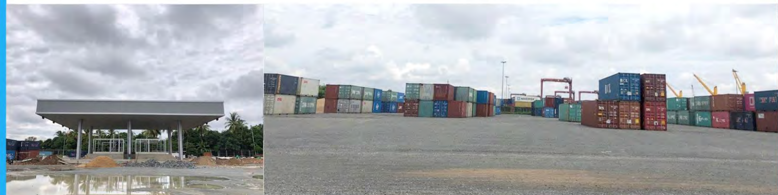
Construction of New Gate
